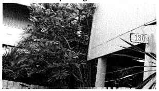
Units 208/210 – Plants growing up the side of the Building. They should be removed or moved away from the building. They will damage the paint and the siding.
